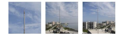
ERICO INTERCEPTOR ESE i-Series generates controlled magnitude and frequency pulses at the tip of the terminal during high static fields prior to a lightning discharge. This enables the creation of an upward leader from the terminal that propagates toward the downward leader coming from the thunder cloud.
