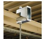
Structural attachment to beams to support threaded rod
