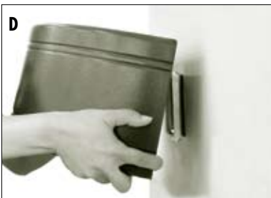
Connect wires and mount fixture to the plate
