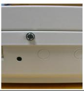
2. APPLY PRESSURE AT LANCE LOCATIONS TO REMOVE THE LIGHT PANEL FROM THE CHANNEL.
