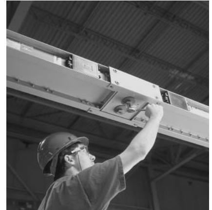
Typical Busway Installation (Torque Indicating Bolt)
