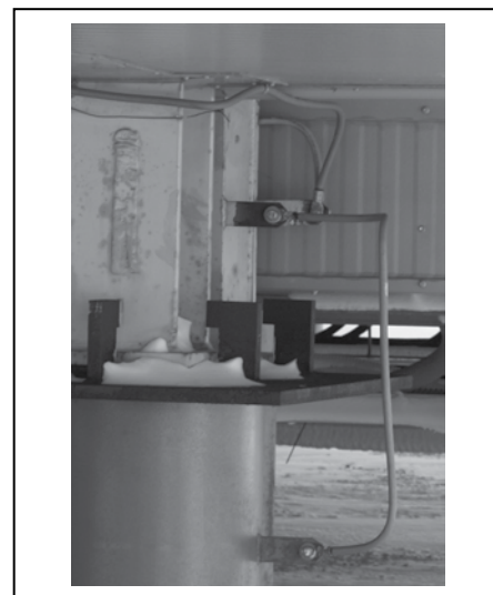
Right: Application image of GROUND TAB used with terminals
