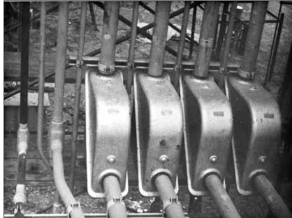
Conduit Systems Installations
